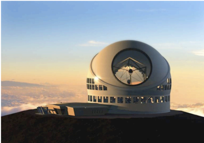
Facility with Calotte Enclosure (Canadian design)
